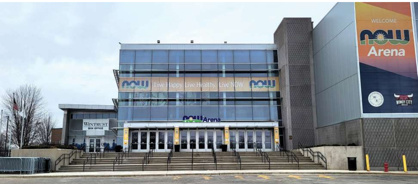
NOW Arena – Main Stair Repair RFP Facilities
