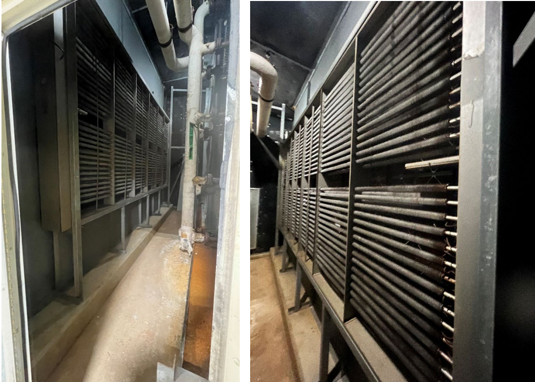
Interior view of existing finned tubes
