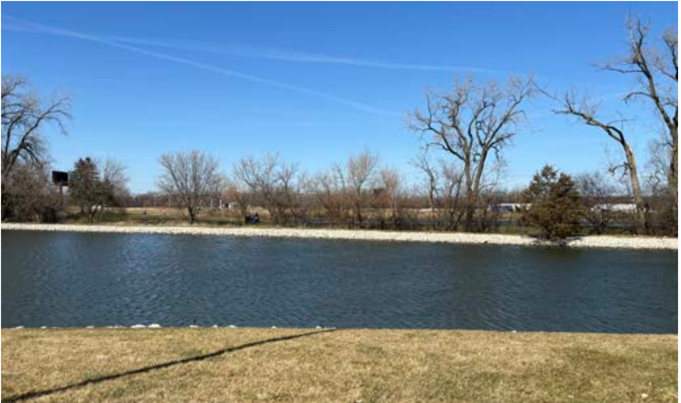
Existing stormwater detention pond at north end of property
