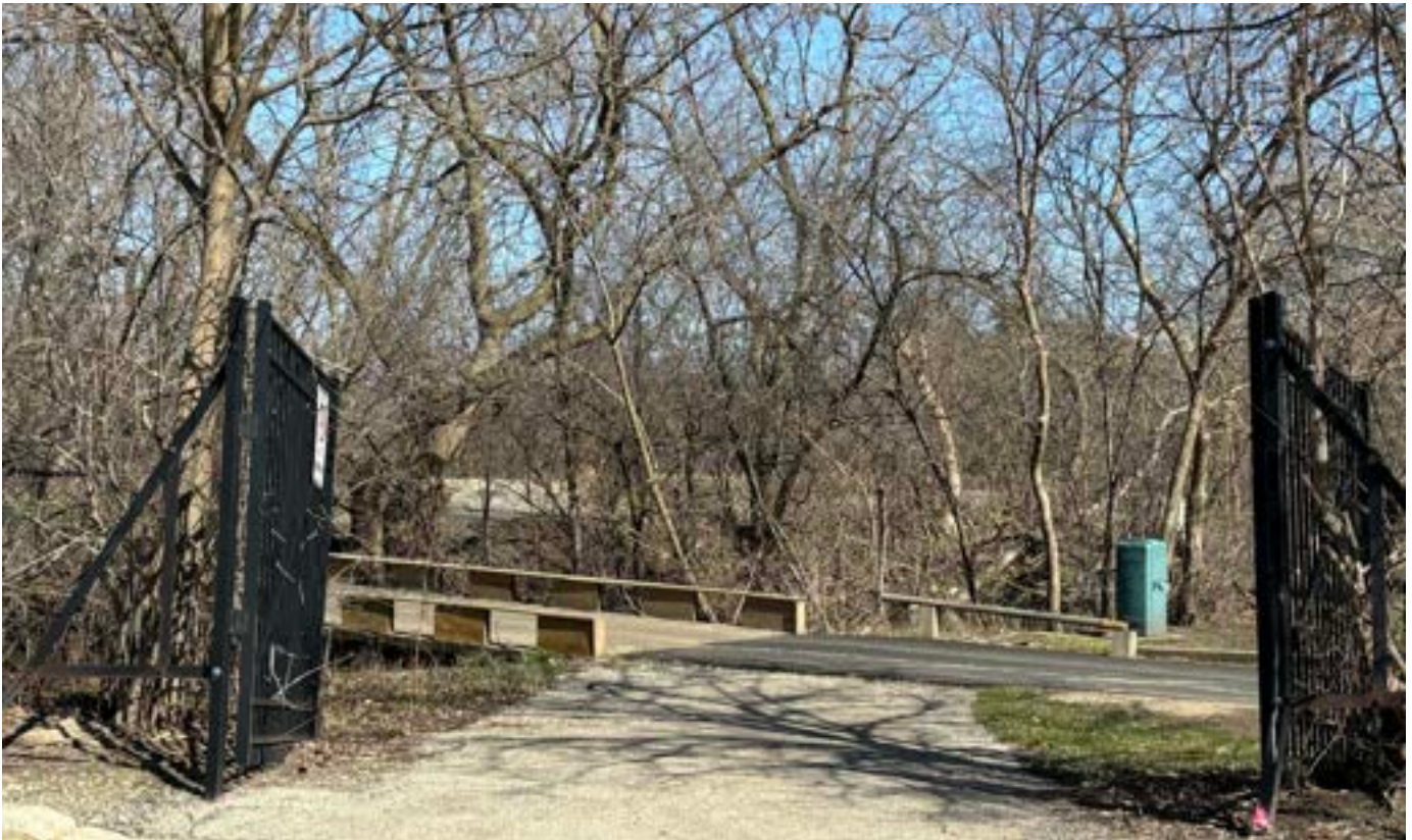
Existing cart path / pedestrian bridge over Poplar Creek
