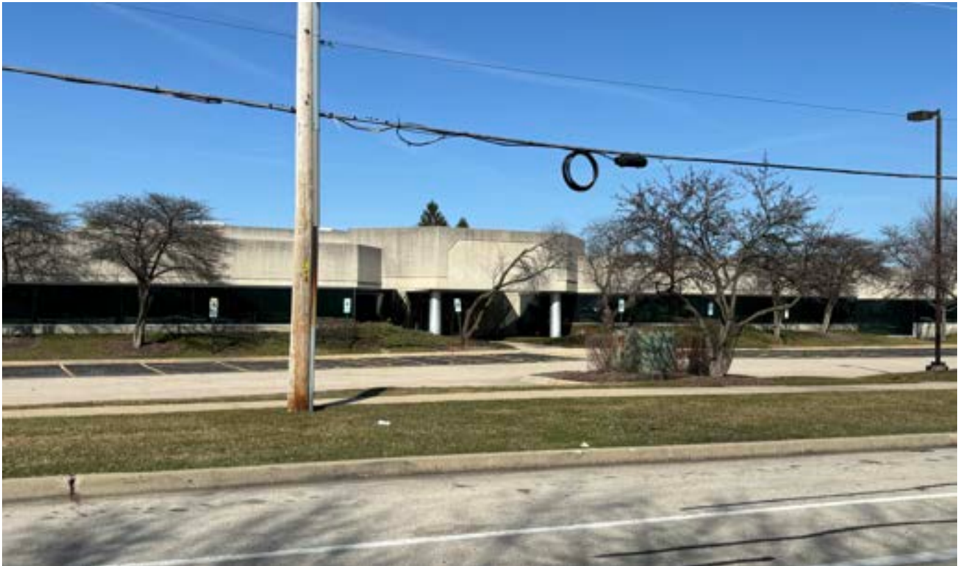
Existing office building on site
