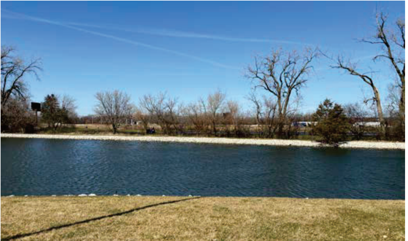
Existing stormwater detention pond at north end of property
