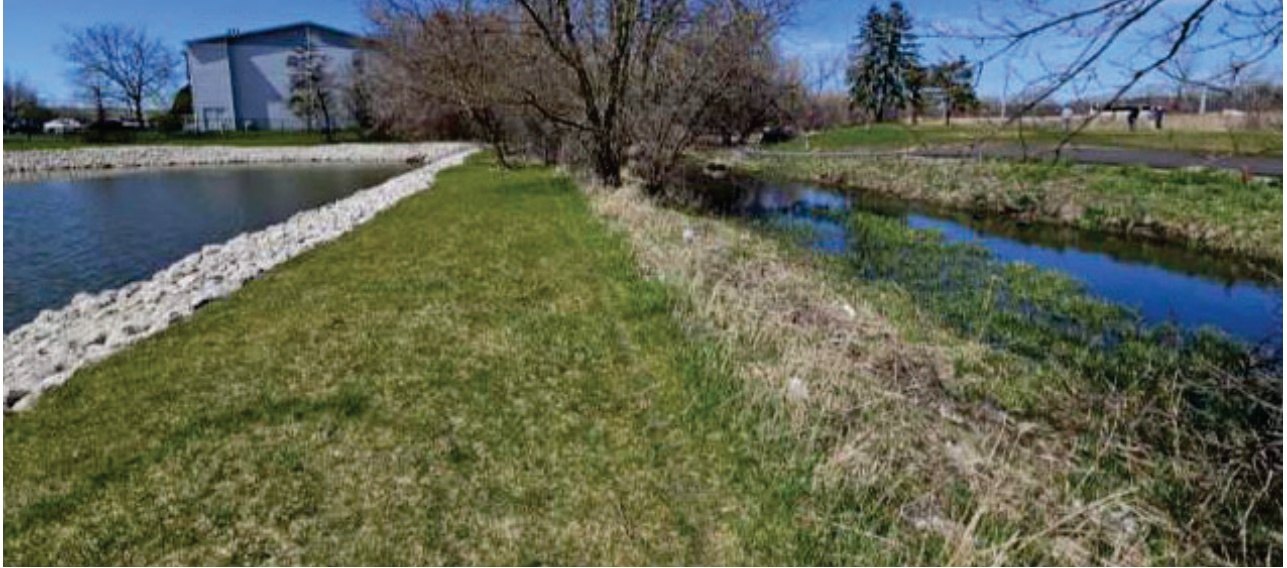
Existing stormwater detention pond at north end of property & Poplar Creek, looking West
