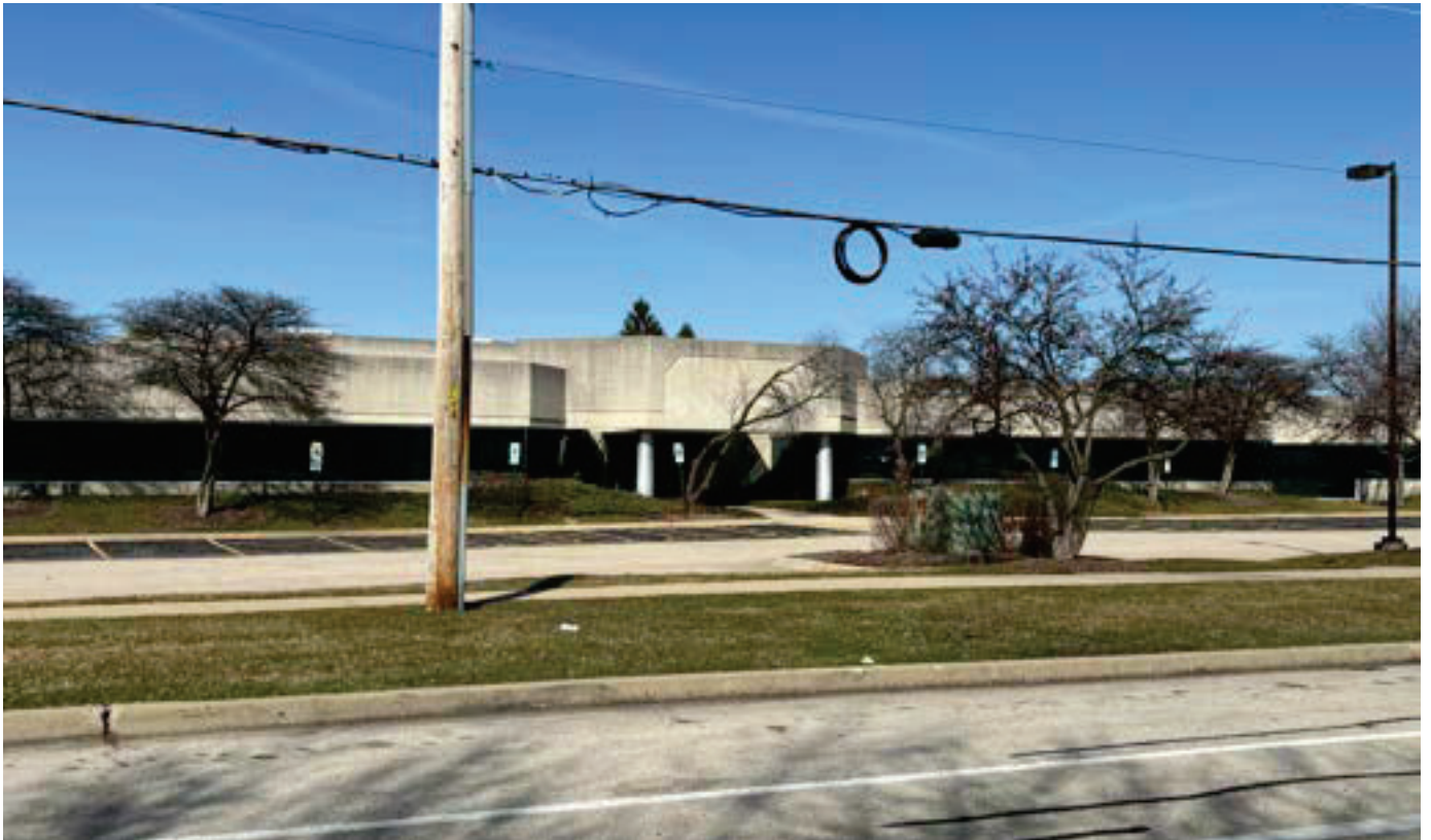
Existing office building on site
