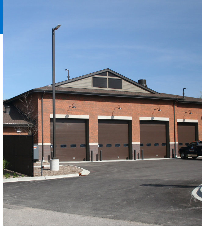
Front Exterior of Public Works Facility
